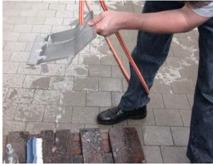
10) Check proper functioning of the filter, water shall pass well.
